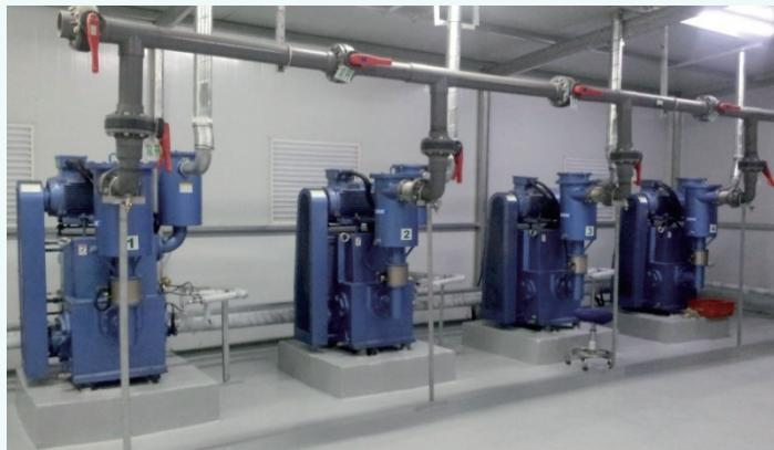
Central vacuum system made by **ELIVAC** piston pump set replaced dozens individual rotary vane pumps that reduced the work place noise level dramatically and made the work area neat.
